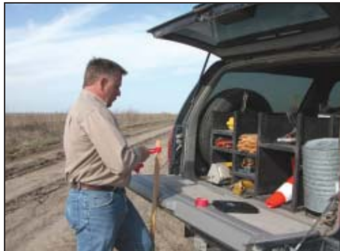
Left: Staking Technician Mark Engler prepares stakes to use when marking where the poles will be set.
